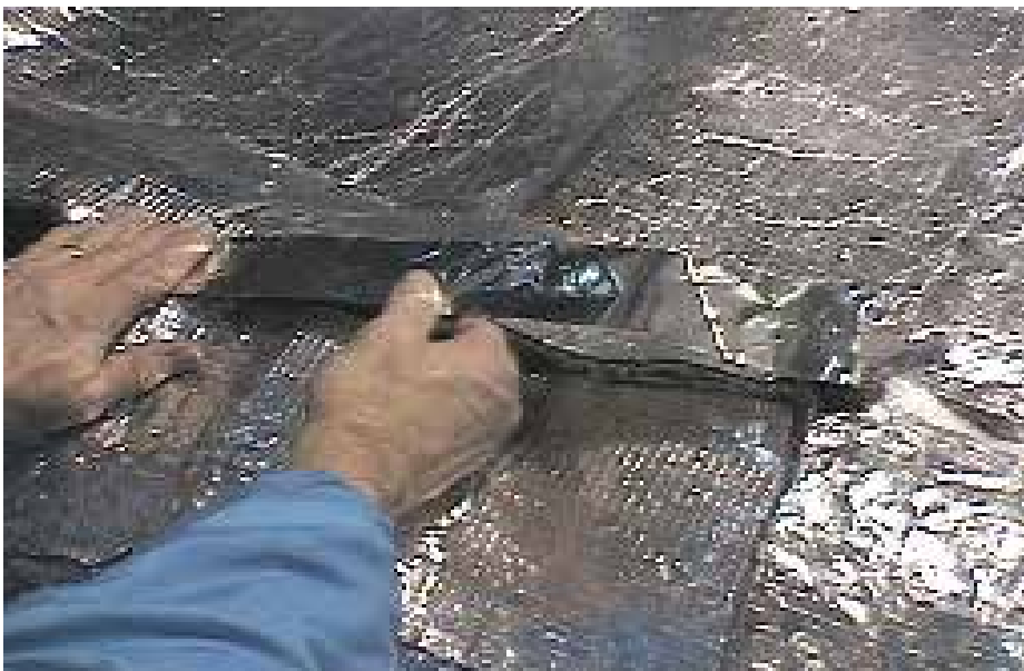
Cowl Absorber Panel ready to tape.
